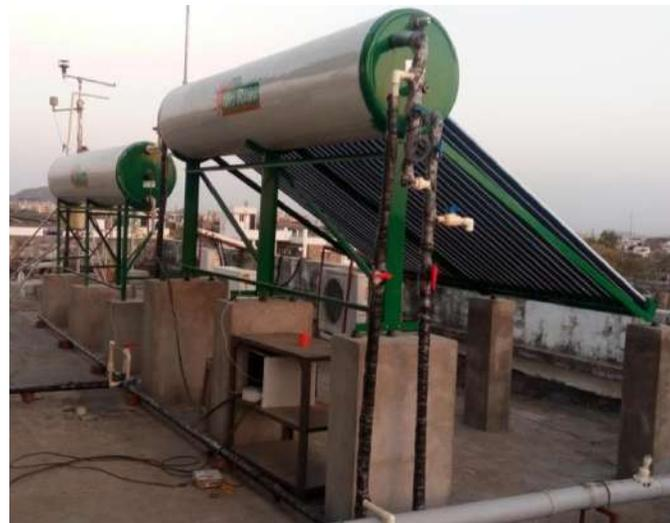
Evacuated tube collectors with buffer tank
