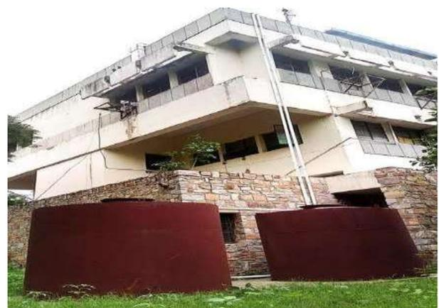
Chilled water based thermal storage
