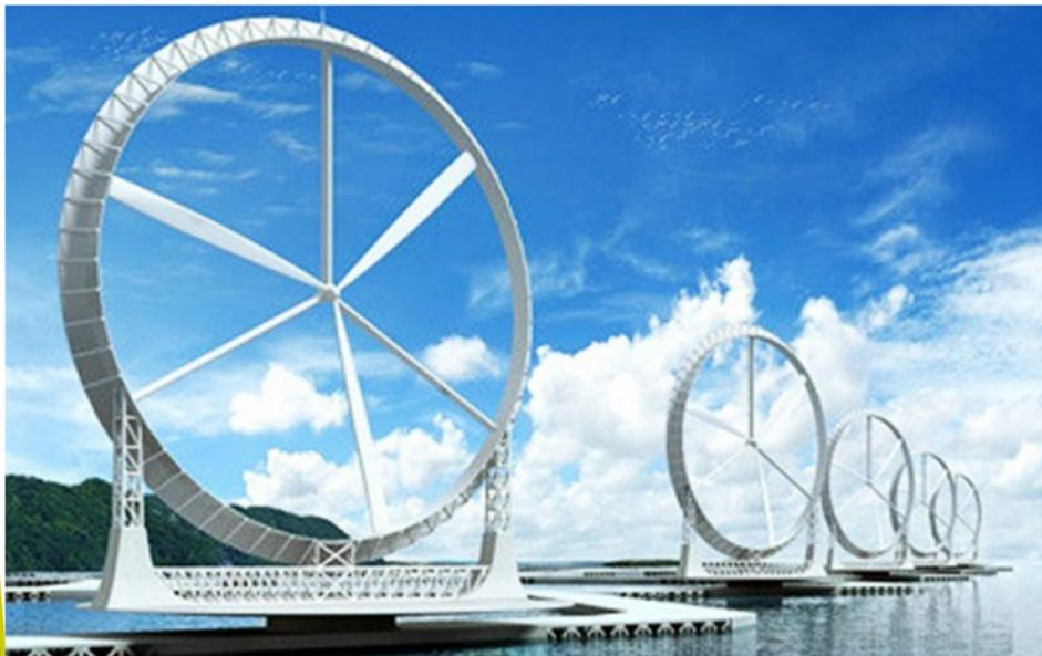
A **wind lens** is a modification made to a wind turbine to make it a more efficient way to capture wind energy. The modification is a ring structure called a "brim" or "wind lens" which surrounds the blades, diverting air away from the exhaust outflow behind the blades. The turbulence created as a result of the new configura-
