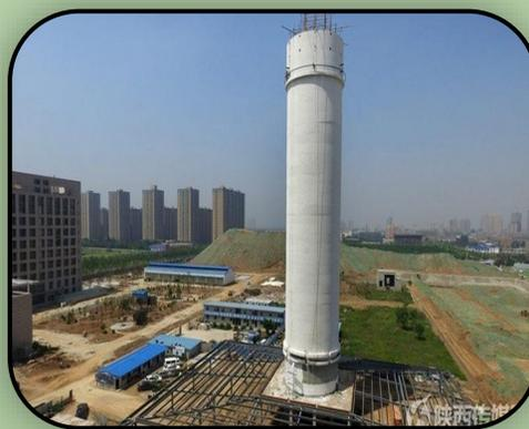
ings on greenhouses enable glass to absorb solar radiation at higher efficiency. According to its original design, the full-sized tower will reach 500 metres high with diameter of 200 metres. This tower size will capture greenhouses in nearly 30 square kilometres and will be capable of purifying the air for small-sized city.
