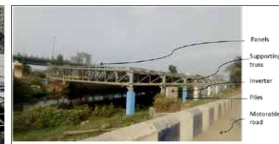
Fig. 4. View from the canal side road of the installed 500kW solar PV plant parts
